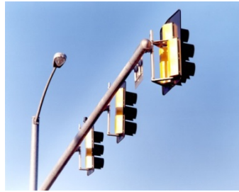
Permanent mast arms
